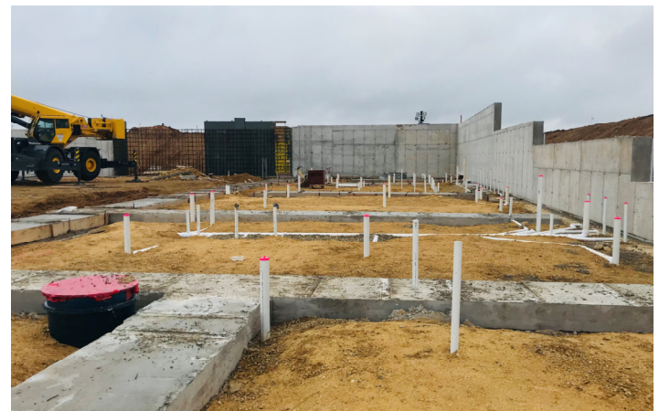
Locker Room Interior Footing & Plumbing Rough-in
