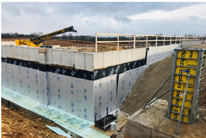
Waterproofing & Backfilling Gym Walls
